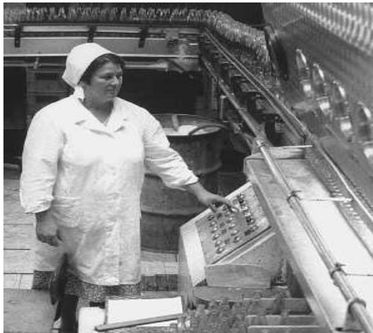
Figure 2: Soft drink canning line showing filling operations
